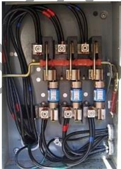
Figure 4-8 A three-phase fused disconnect switch. In order to ensure proper equipment operation, all wiring connections must be tight and the clips that hold the fuses must be in good condition. When removing fuses from a disconnect box the proper method is to use a fuse puller rather than a screwdriver to pry them loose.
