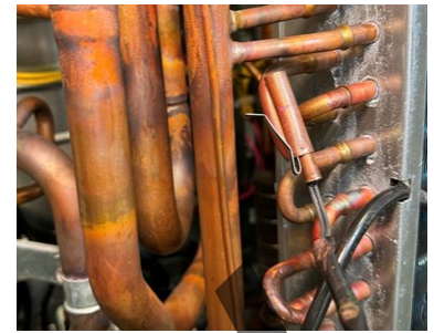
Figure 2-12. A heat exchanger thermistor.
