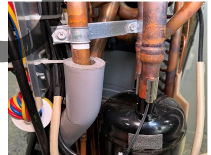
Figure 2-14. Suction line thermistor.
