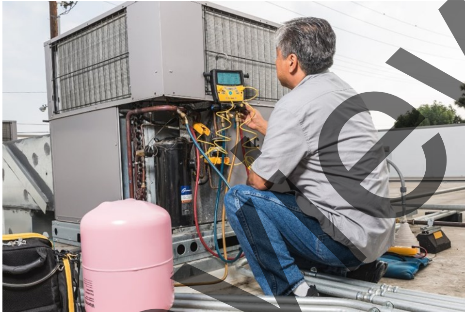
Figure 9-11. Charging of ALL inverters is specific to the equipment being installed. Always refer to the installation manual for proper charging design and additional refrigerant charge (if applicable).
