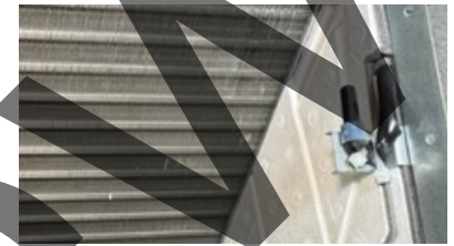
Figure 2-13. Return air temperature thermistor.
