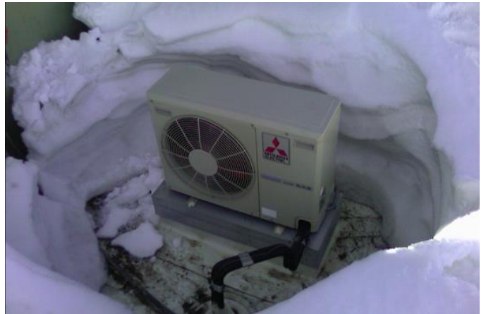
Figure 7-20 A server room condenser placed adjacent to a warehouse wall on the leeward side of the building which concentrated the snow in this exact spot. After several large storms, the condenser was enclosed inside a cave of snow and ice. Less than 10 feet away, the snow was only a few inches in depth. Location, location, location!
